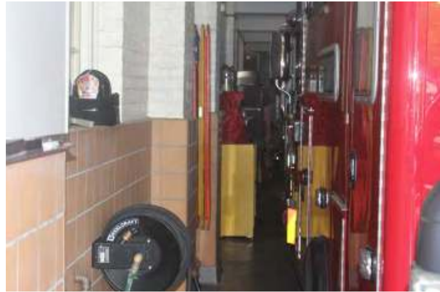
Not enough space to open equipment and maintain/clean properly
