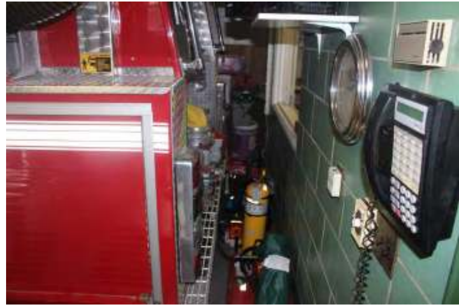
Apparatus against rear wall (zero clearance)
