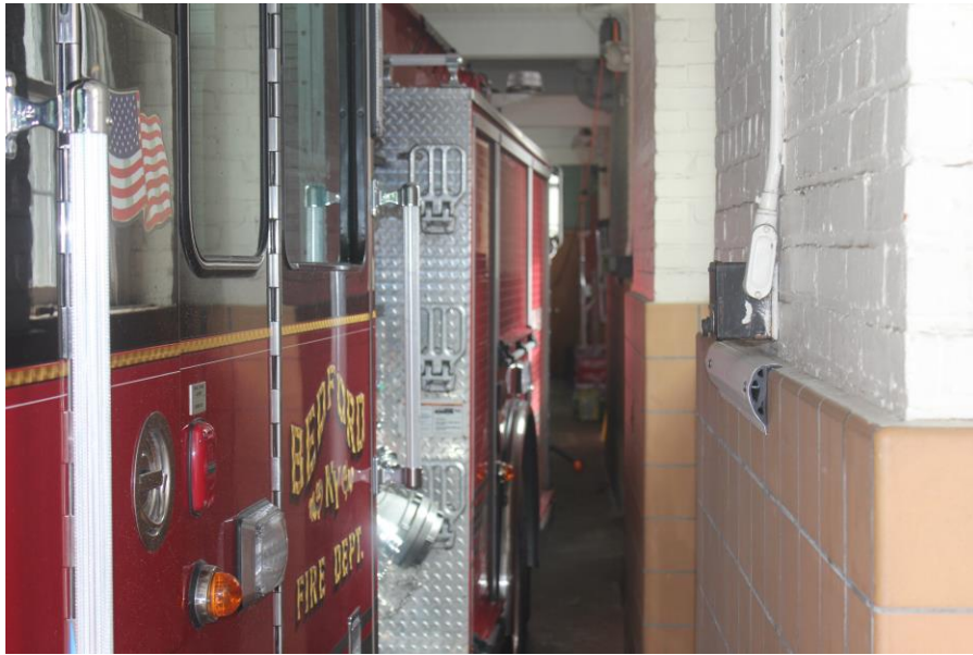
Not enough space to open vehicle doors
