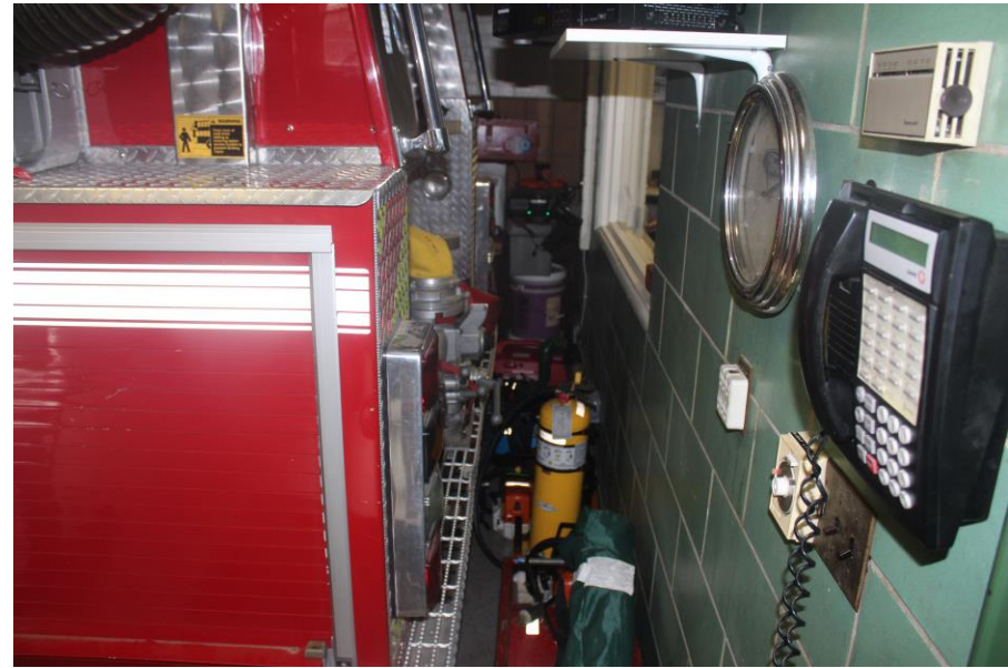
Apparatus against rear wall (zero clearance)
