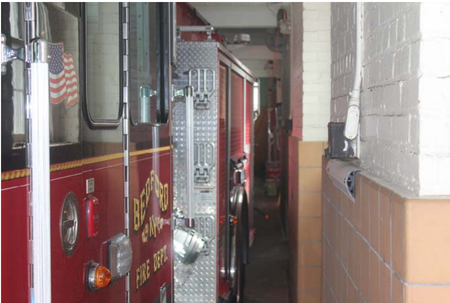
Not enough space to open vehicle doors
